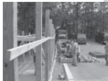
Pi Kappa Phi members building the covered walkway
