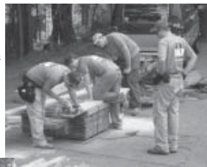
Volunteers measuring and cutting wood for the covered walkway
