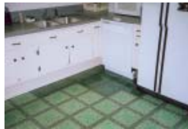
East Hembree cabinets and flooring to be replaced
